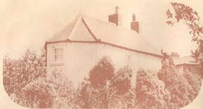
The old lock-keeper's house, with half-octagonal end, where the excellent visibility from the angled windows enabled the lock-keeper to see all movements on the locks from his living quarters.
