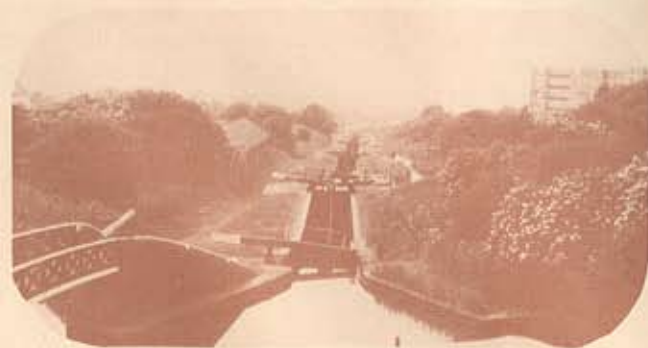
View down the Locks, from Nine Locks Bridge. In the foreground is the roving bridge, a protected structure as are the locks themselves. On the roving bridge parapet can be seen rope marks where generations of horses hauled boats up and down the locks.
