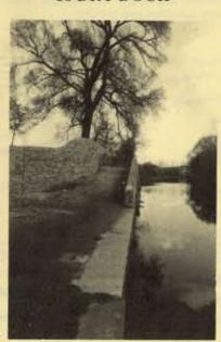
The wooden narrowboats that served the Ironworks were probably built and repaired here, and in fact the old workshops, now in ruins and with an early iron roof structure can be seen to the rear. A large anvil was set in part of the workshops, confirming their role. Water flow into or out of the Dry Dock was controlled by a system of sluices.
