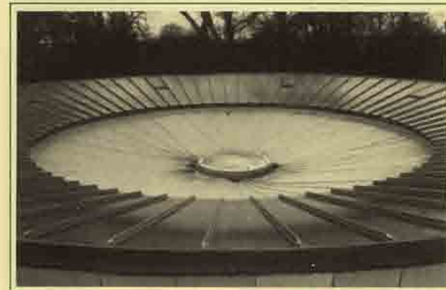
Tropical Bird House; roof detail
