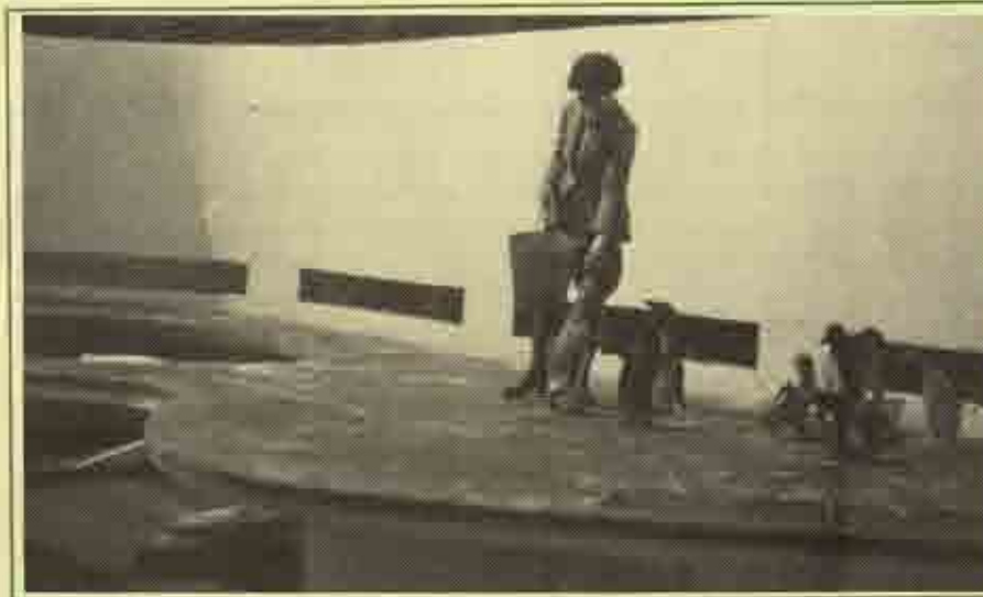
The Penguin Pool before demolition
