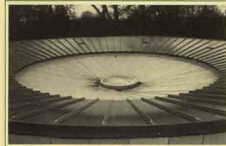
Tropical Bird House; roof detail
