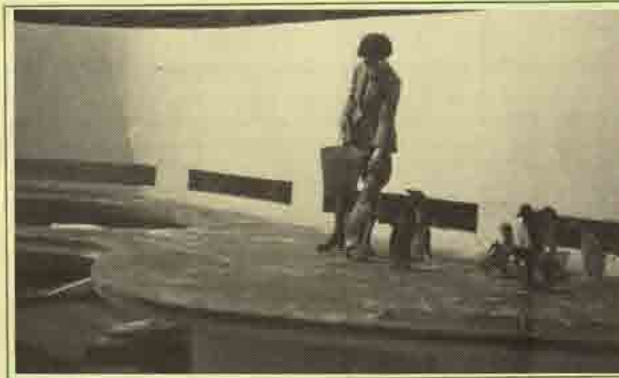
The Penguin Pool before demolition
