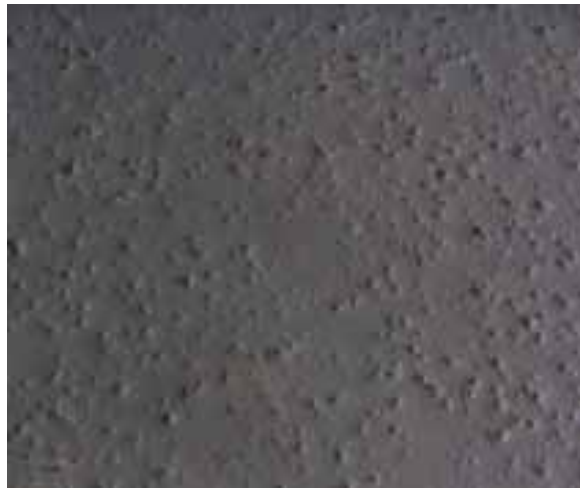
Figure 21 - Resin & Aggregate Surface
