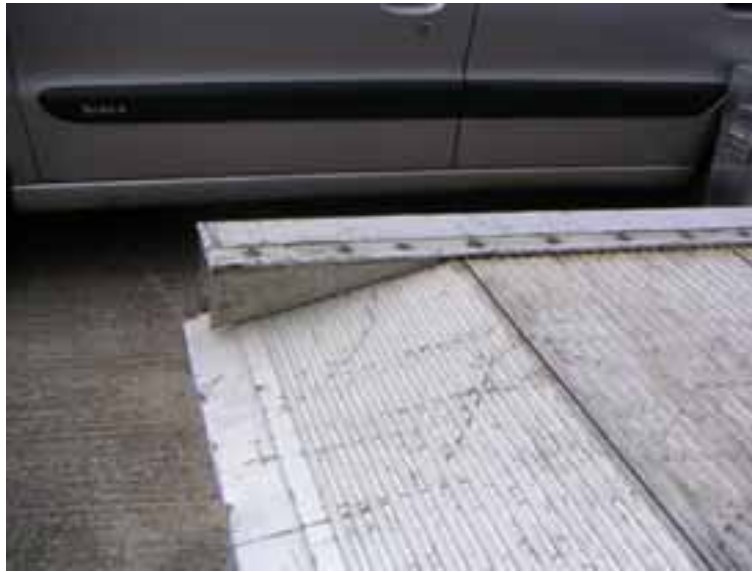
Figure 6 – Tail lift design that could result in a trip.
