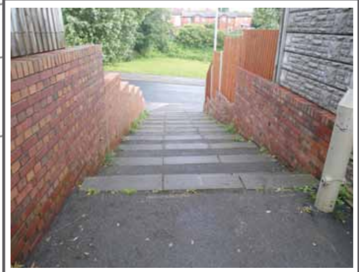
Improve PROW signage and tactile paving
